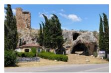
The tower has an almost square base, measuring 7.8 by 7.9 meters, with walls 1.65 meters thick at the base. It is preserved to a height of around 15 meters. The structure is built with hewn stone, mostly undressed but arranged in relatively regular courses, with dressed stones used for the quoins. Some of these dressed stones are spolia, repurposed from the nearby acropolis of ancient Haliartos. The size of the stones diminishes with height.
